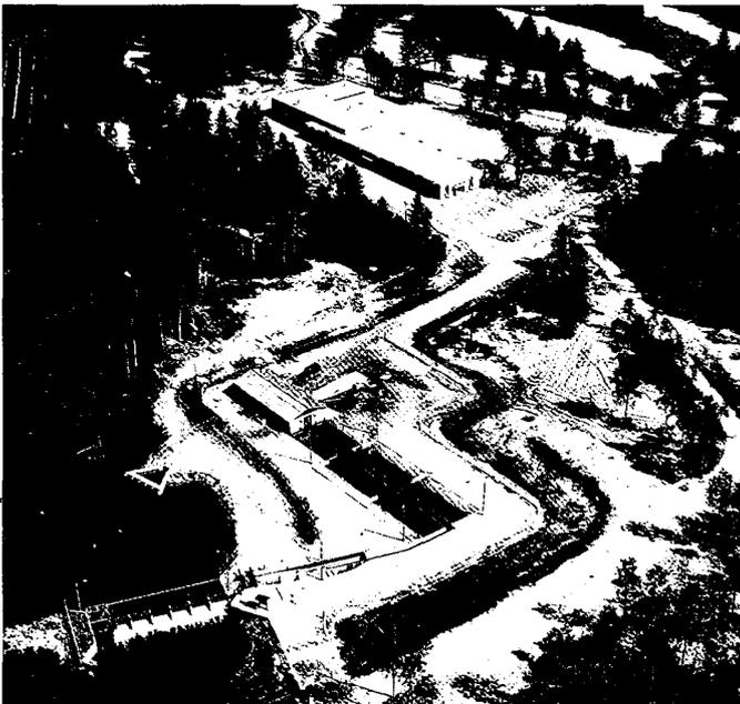
Upper Platte River weir (lower left), fishway, holding ponds and egg taking station with new hatchery building (top center).
