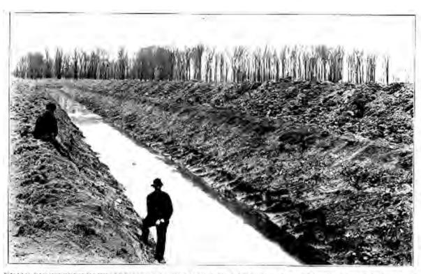
DRAIN EIGHT FEET BOTTOM WIDTH, EIGHT AND ONE HALF PEET DEEP, CONSTRUCTED BY DREDGE SHOWN IN PLATE V. IN 1917, AT COST OF \$7.25 FER ROD ABOUT \$4845 PER CUBIC YARD! TO REPLACE SHALLOW TEAM AND SCRAPER DRAIN CONSTRUCTED IN 1914 AT A COST OF \$1.00 PER ROD.
