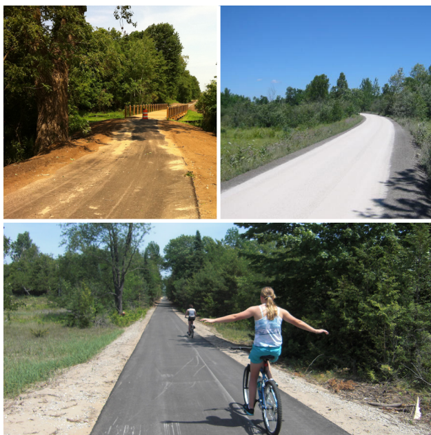
Improved trail surfaces, clockwise: base course of asphalt trail, limestone trail, asphalt trail
